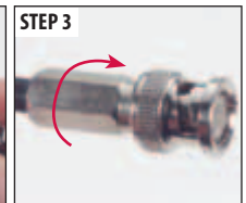
STEP 3 Twist connector body onto cable.
