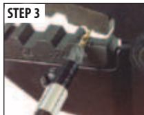
STEP 3 Slide pin onto center conductor making sure base of pin meets dielectric. Crimp in place.
